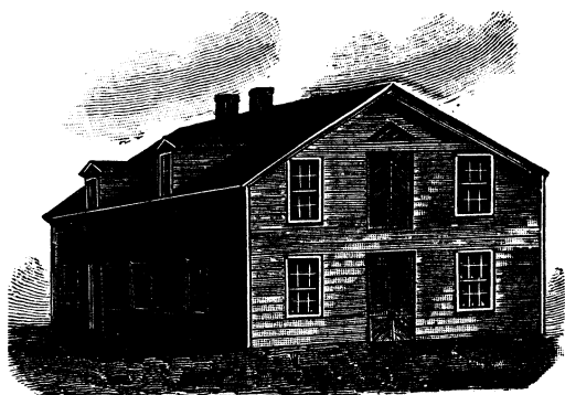
THE OLD YELLOW WAREHOUSE—BUILT IN 1834—TORN DOWN IN 1889.
